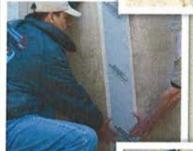
We apply hydrophobic gel on the back of the Techni-Crack\* membrane and apply it to the wall. We then tie it into the Water Trek Aqua Route\* system or drywell.
