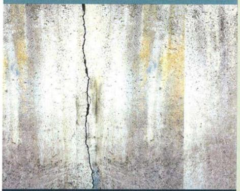
Poured foundation wall cracks generate water onto the basement floor.
