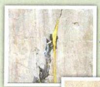
Optional polyurethane injection stops water from the outside of the wall (for really severe leaks).
